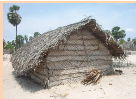
One of the women's temporary houses in Jaffna made with Palmyra leaves. Still many people live in this kinds of temporary houses.
